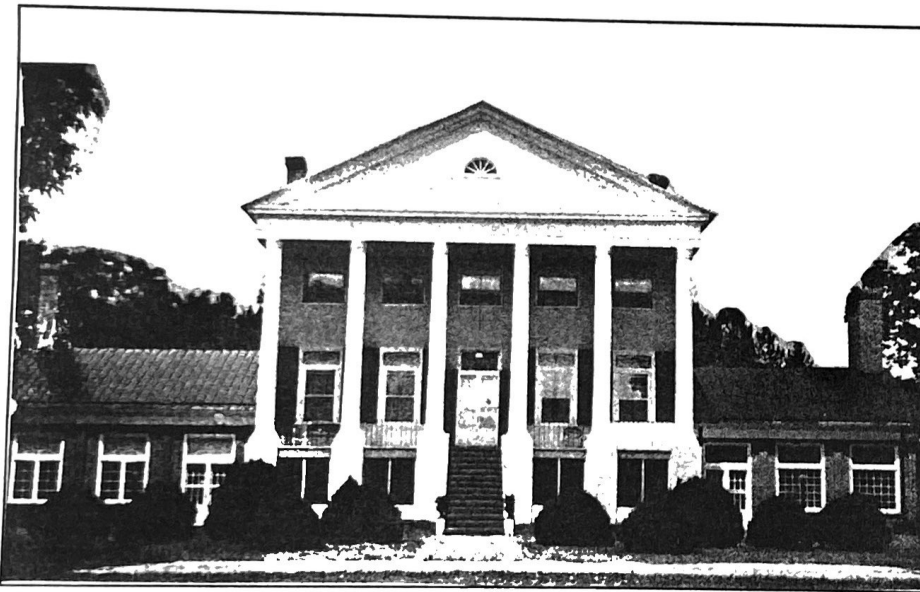
Figure 37 Ingleside, as it appears today.
